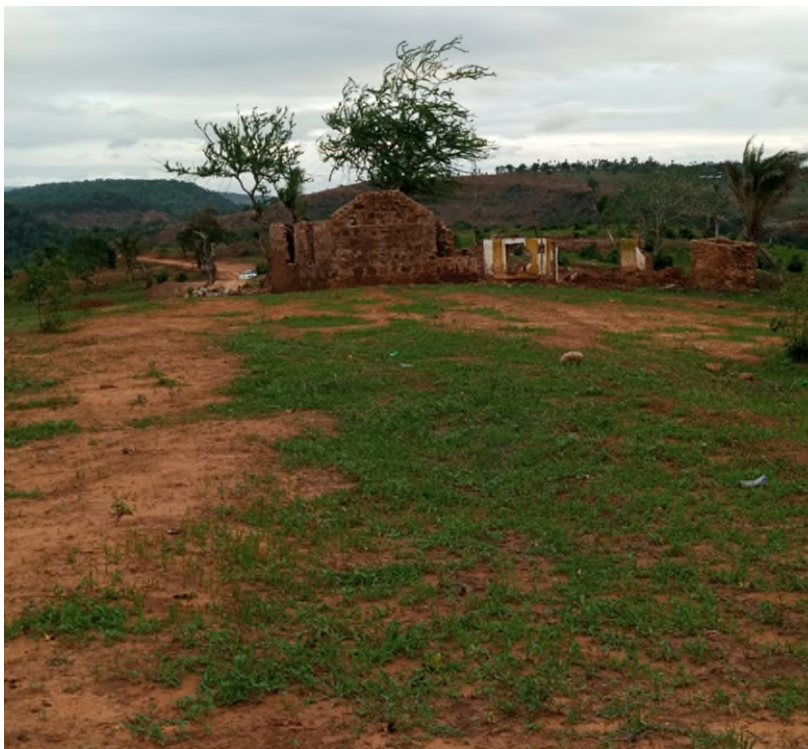
Figure 2 : Photos of selected WTP site
